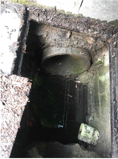
Photo 8 (looking into CB #4): Type 1 Catch Basin (#4). 12" concrete outlet flowing N.
