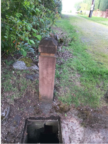
Photo 12 (looking into CB #7): 12" concrete outlet flowing N.
