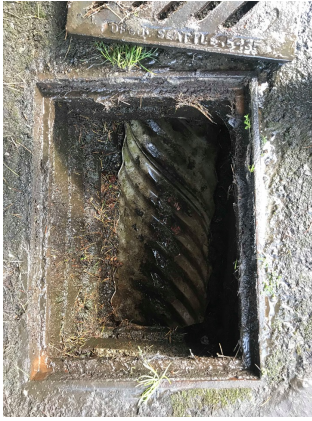
Photo 6 (looking into CB #3): Type 1 Catch Basin (#3). 12" concrete outlet flowing N.
