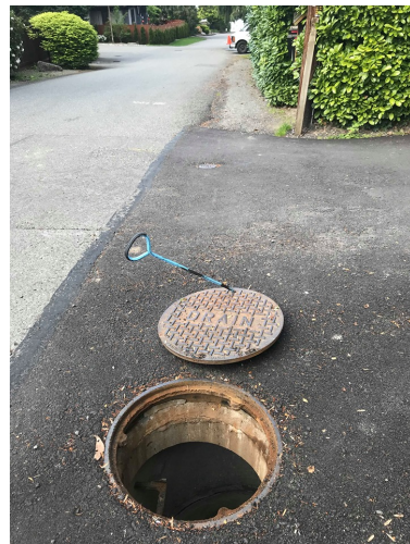
Photo 4 (looking N): Type 2 MH (#2). Inlet from 8" corrugated pipe.
