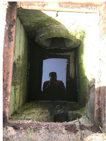
Photo 17 (looking into CB#9): Type 1 CB (#9). 12" concrete pipe outlet flowing north.
