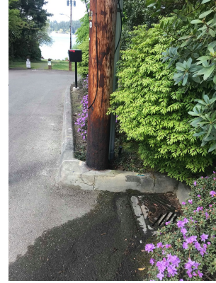
Photo 7 (looking N): Type 1 Catch Basin (#4). 12" concrete inlet.
