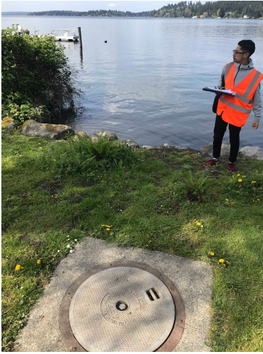
Photo 18 (looking N): Manhole (#10) that outflows into Lake Washington.
