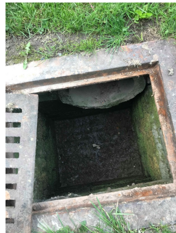
Photo 15 (Looking N): Type 1 Catch Basin (#8). 12" concrete inlet.
