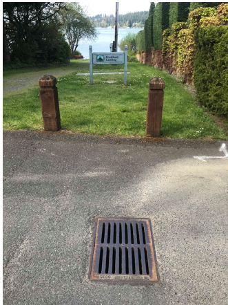
Photo 10 (looking N): Type 1 Catch Basin (#6). 12" concrete inlet.
