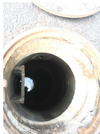
Photo 5 (looking into MH #2): Type 2 Manhole (#2). 12" concrete pipe outlet flowing N.
