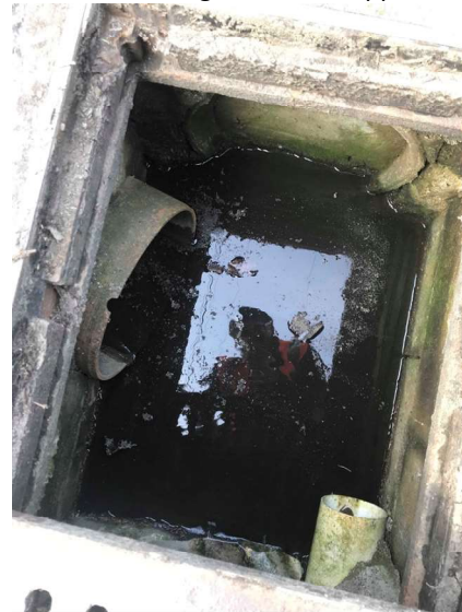
Photo 11 (looking into CB #6): 12" concrete outlet flowing W.
