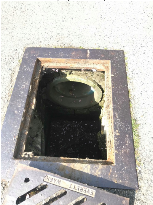
Photo 3 (looking into CB #1): Type 1 Catch basin (#1). 12" concrete pipe outlet flowing N.
