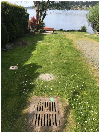
Photo 16 (looking N): Type 1 Catch Basin (#9). 12" concrete inlet.
