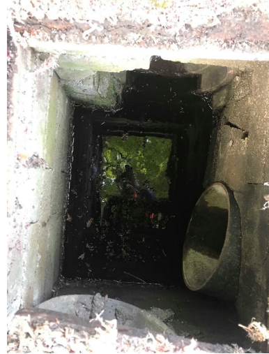
Photo 13 (looking N): Type 1 Catch Basin (#7). 12" concrete inlet.
