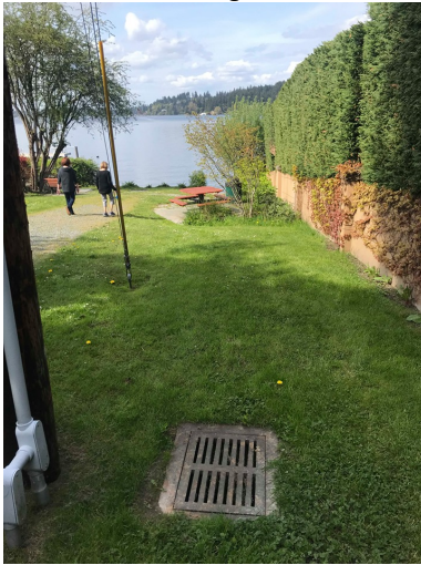
Photo 14 (looking into CB #8): Type 1 Catch Basin (#8). 12" concrete pipe outlet flowing NW.
